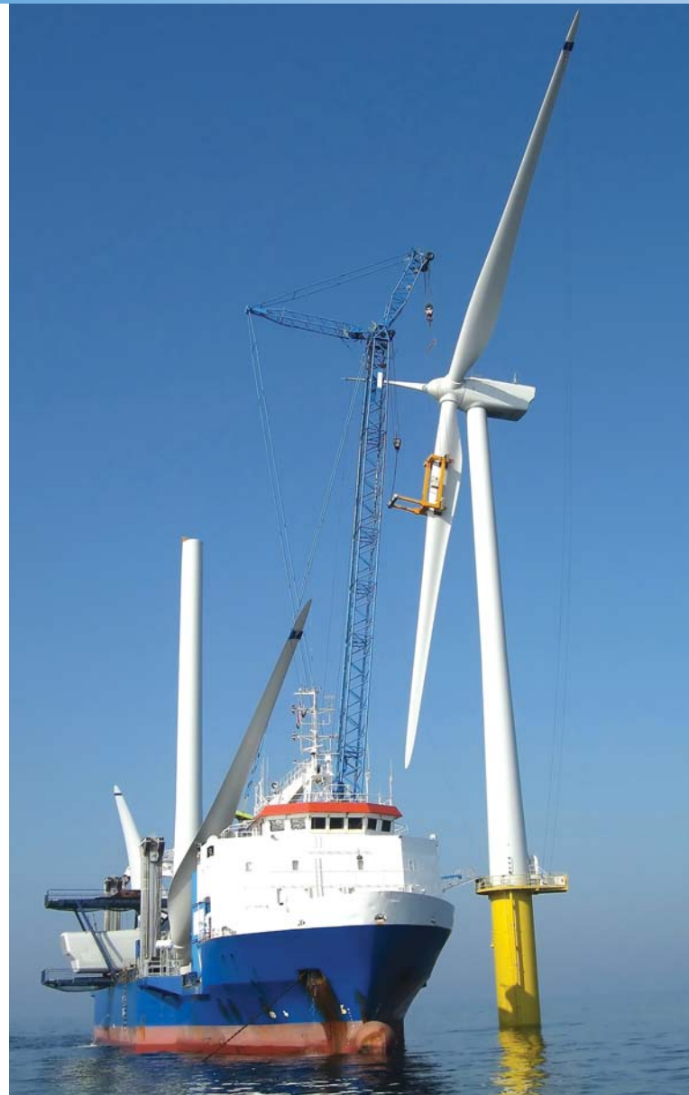
Installation of an offshore wind turbine
